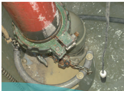
Building site pumps
